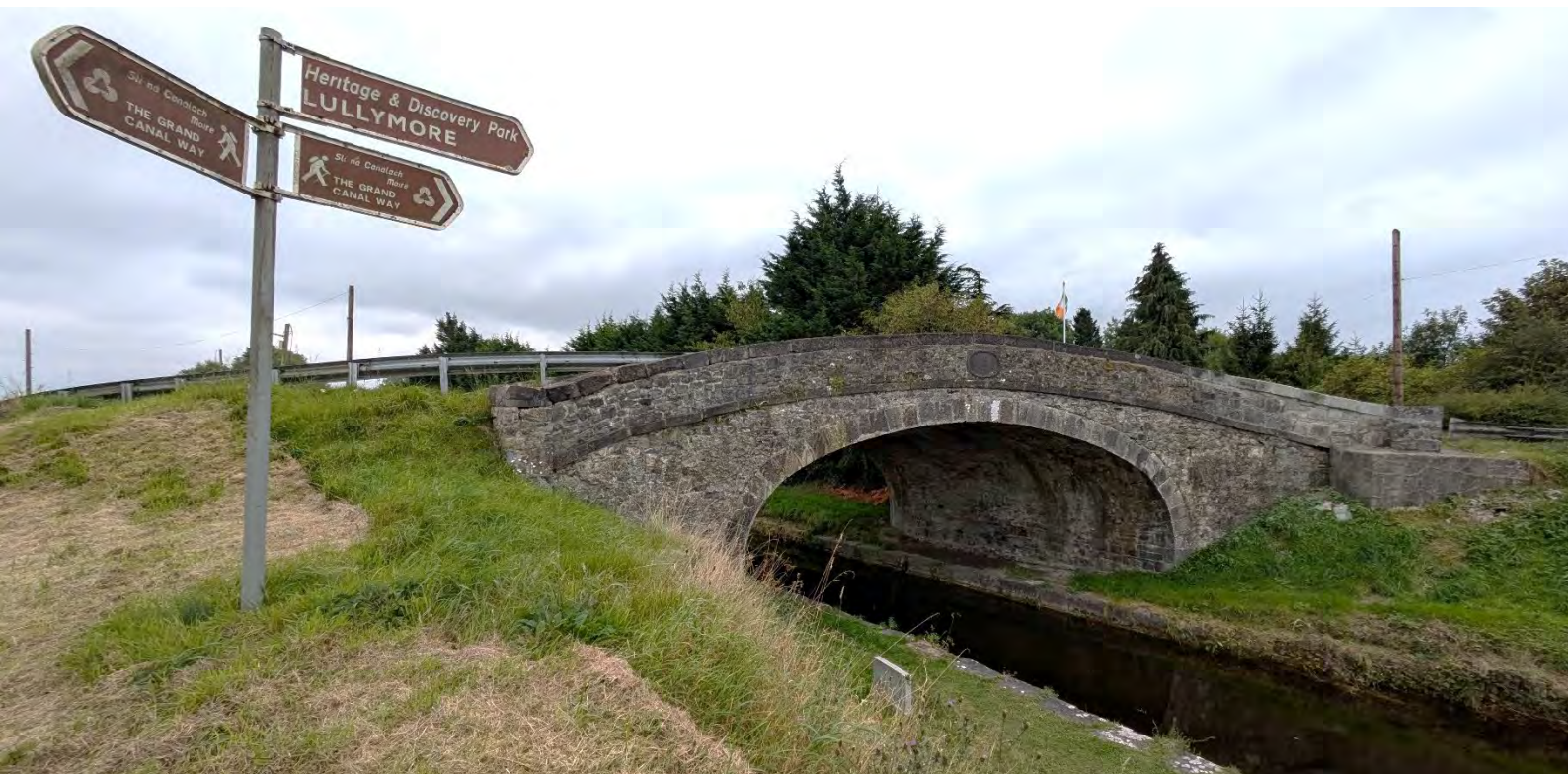
PHOTO 4- 9 GRAND CANAL WEST OF ALLENWOOD
