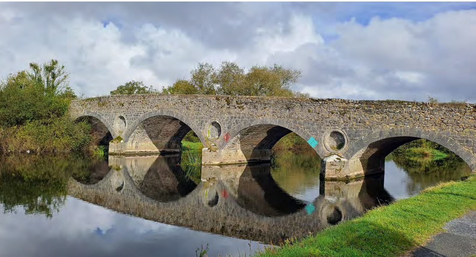
PHOTO 2-8 MAGANEY BRIDGE, FIVE-ARCH LIMESTONE ROAD BRIDGE OVER RIVER BARROW, C. 1800,
